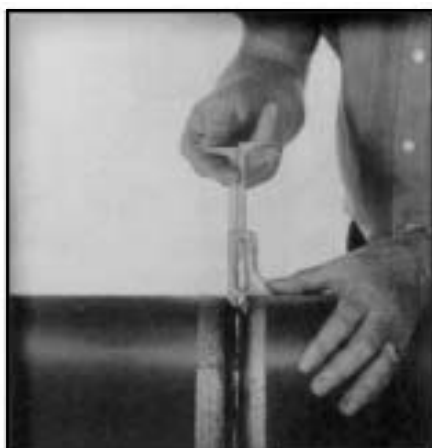
Measure internal mismatch, pipe wall.
